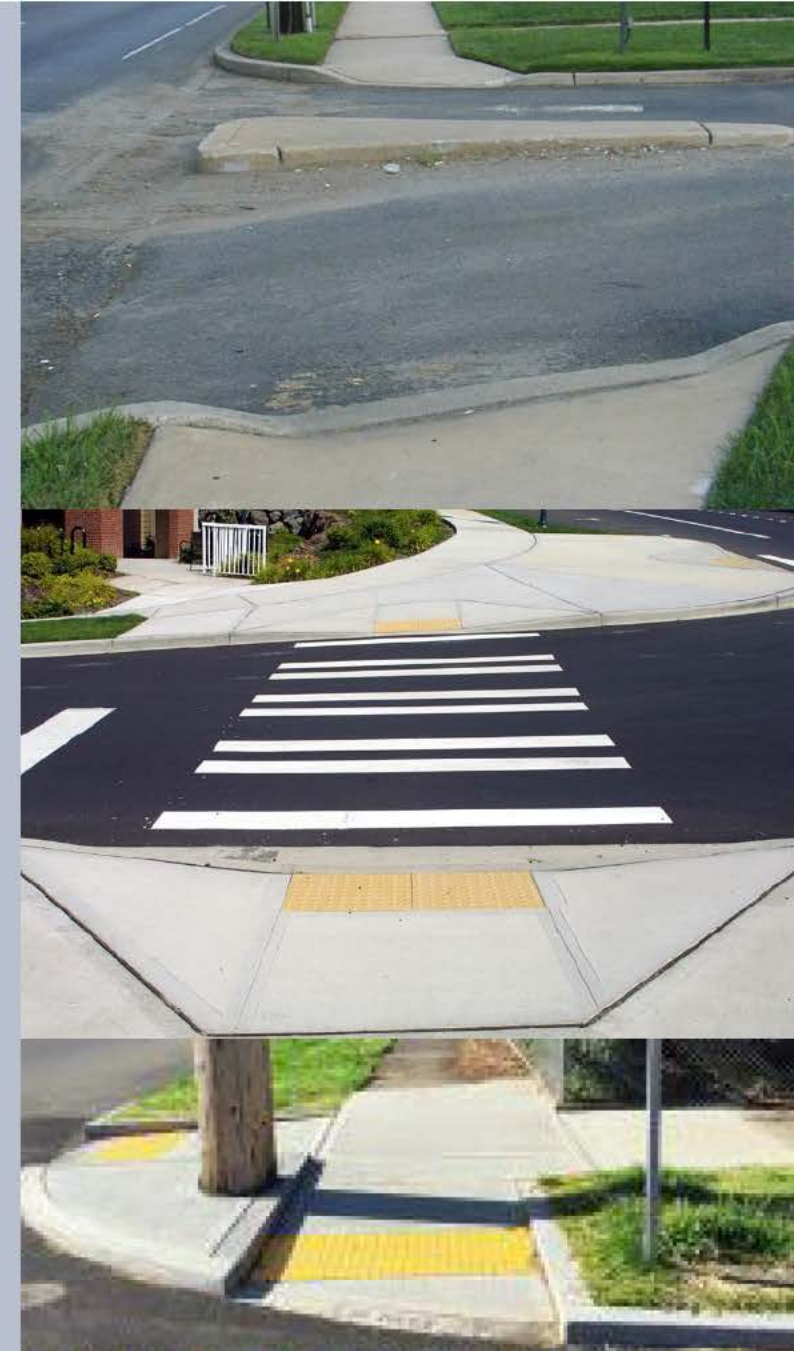
ADA Curb Ramp Improvement Example in Arnada Neighborhood
